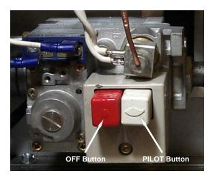
2. Place a flame near the pilot assembly, push and hold the PILOT (white) button in, light the pilot, and continue to depress the button for at least 60 seconds after the pilot lights. Failure to hold the button in long enough will cause the pilot to go out when the button is released. If the pilot goes out when the button is released, wait at least 5 minutes then repeat this step.
